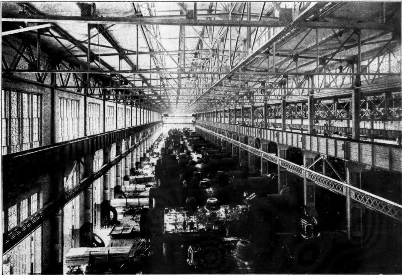
Interior of Erecting Shop. Springfield, Mo., Shops of the Frisco System.
